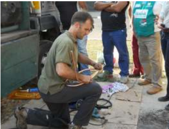
Above: Bending copper loop to fit into tank
